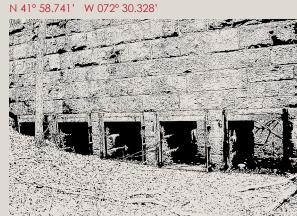
This enormous dam once held back the Scantic to supply power to a dozen mill buildings along its raceway and canal. The raceway section of the dam begins here and flows about half a mile downstream.
