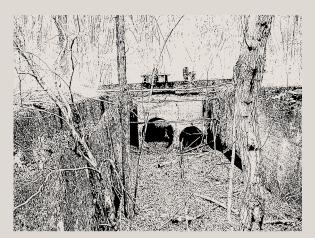
The large openings at the base of the raceway give an indication as to how much water flow was used to power the hydraulic ram. The large raceway was a water storage area that fed the mills in the Scitico powder works. Walking along it can give some idea of the scale of this facility.
