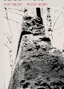
A cross section of the dam can be observed near the river. The dam is constructed of concrete and large stones. It is thick at the bottom and tapers to be more narrow at the top. This was to withstand the variable pressure of the water depth. Deeper water exerts more pressure on the structure, therefore, more strength was needed at the bottom of the dam.
